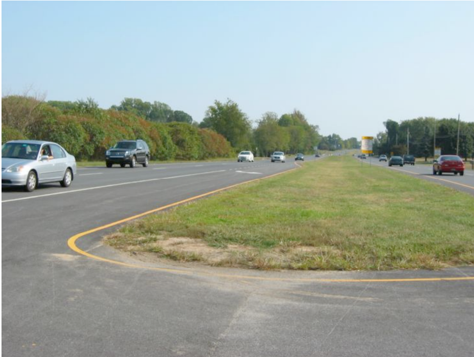
Turning lane at a cross over
